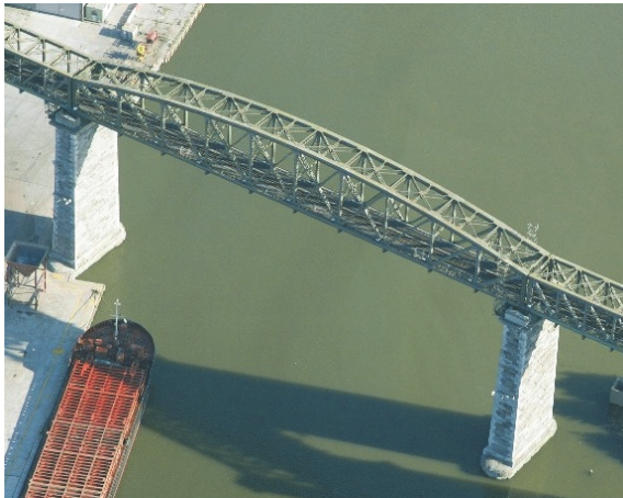
Figure 6: Central span of the Boyne Viaduct, Drogheda, Co. Louth, Ireland.
