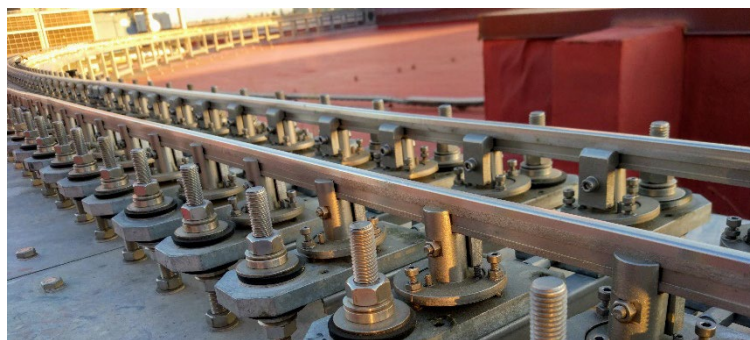
Figure 1. Scaled railroad track located at the University of Seville.
