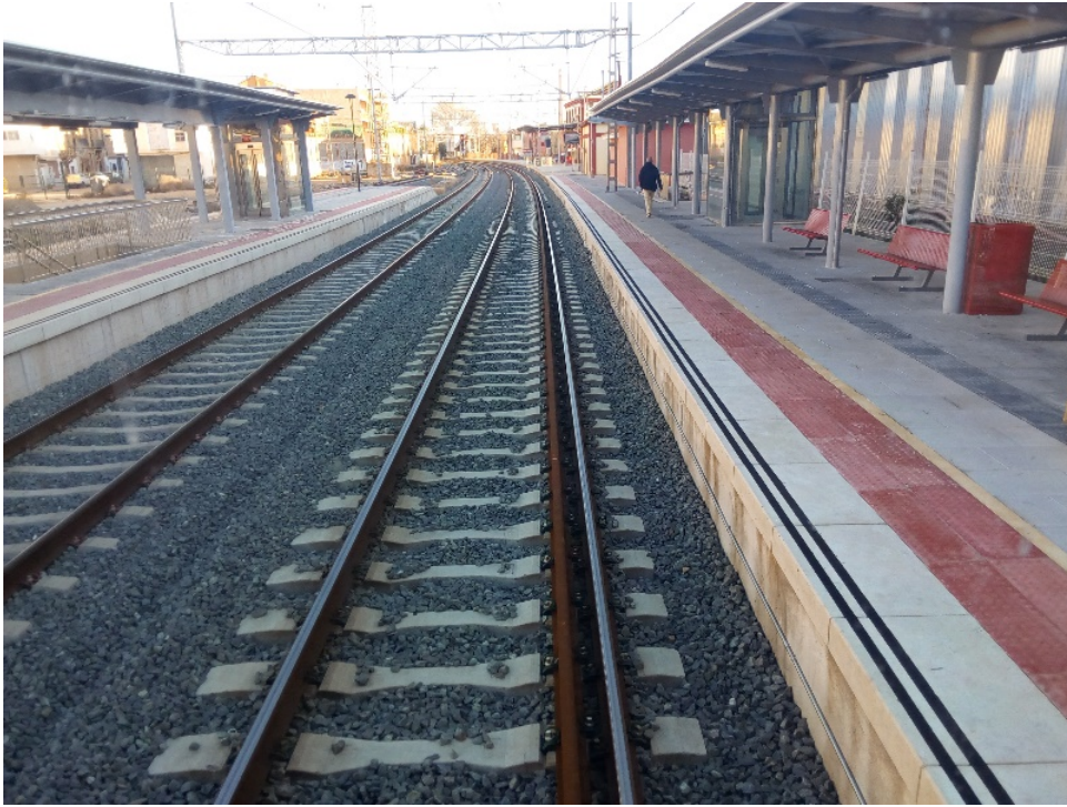
Figure 1: Dual gauge track in Spain.
