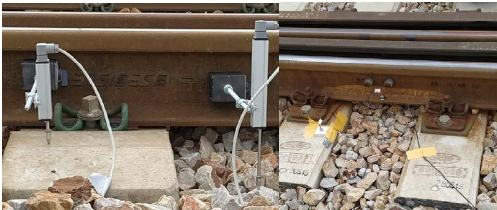
Figure 4. Displacement (right) and accelerometers (left) sensors.
