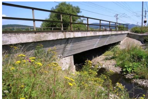
Figure 1: View of the short-span bridge on ŽSR line Žilina – Čadca.
