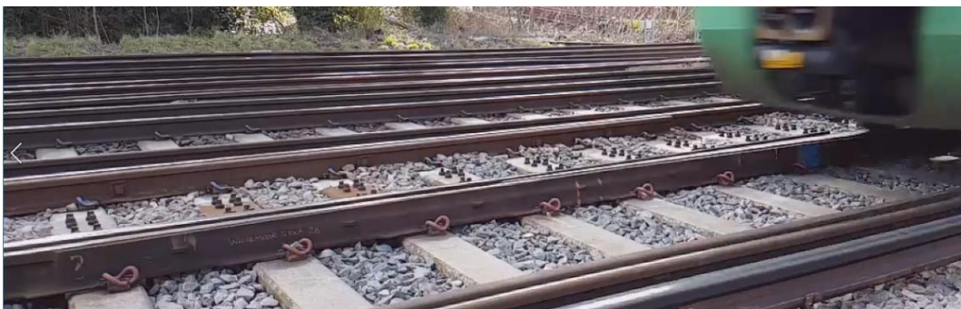
Figure 1: a railway cast manganese crossing under traffic
