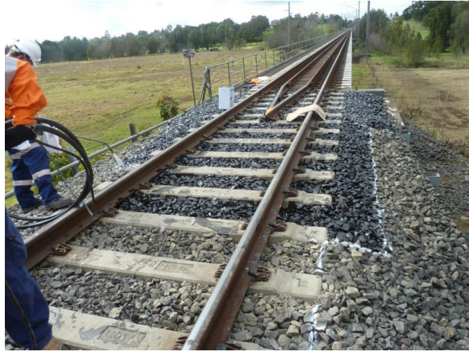
Figure 12: Ballast glue work at the end of the bridge
