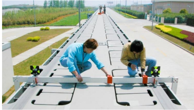
Figure 6: Using Long-wave Set to Measure the Girder Alignment Manually
