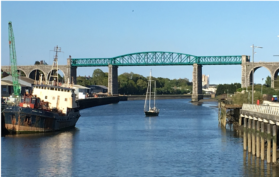
Figure 1: Boyne Viaduct near Drogheda, Ireland. Photo by R. Loendersloot.
