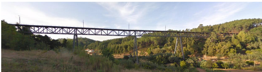
Figure 6: General view of the Várzeas Bridge
