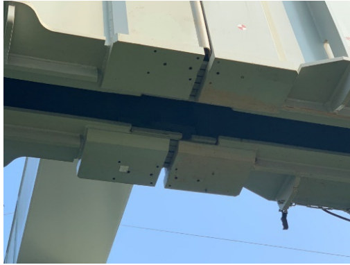
Figure 6: Steel box girders.
