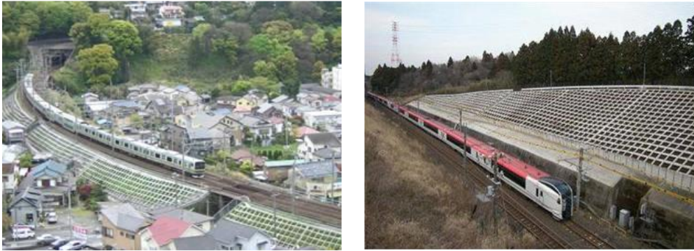
(a) Embankment slope protection works (b) Cut slope protection works
