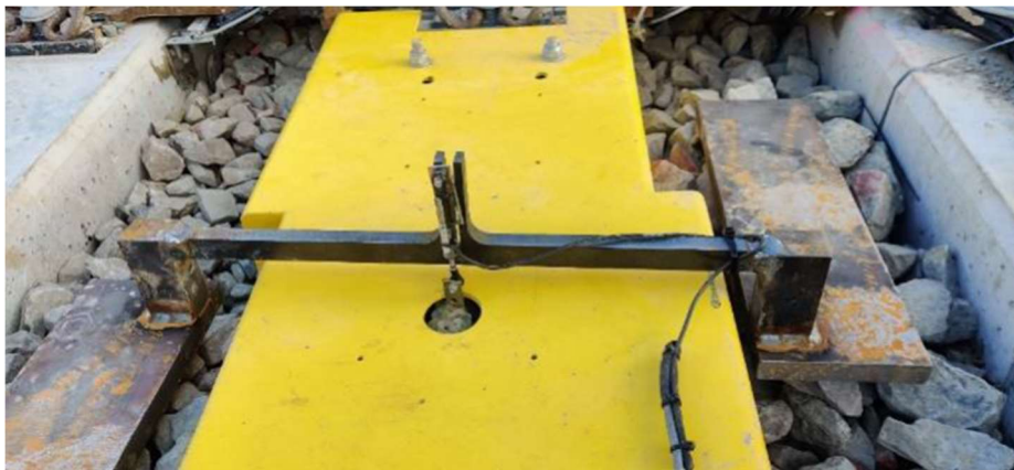
Figure 4: Installed sleeper displacement sensor to measure the ballast deflection.
