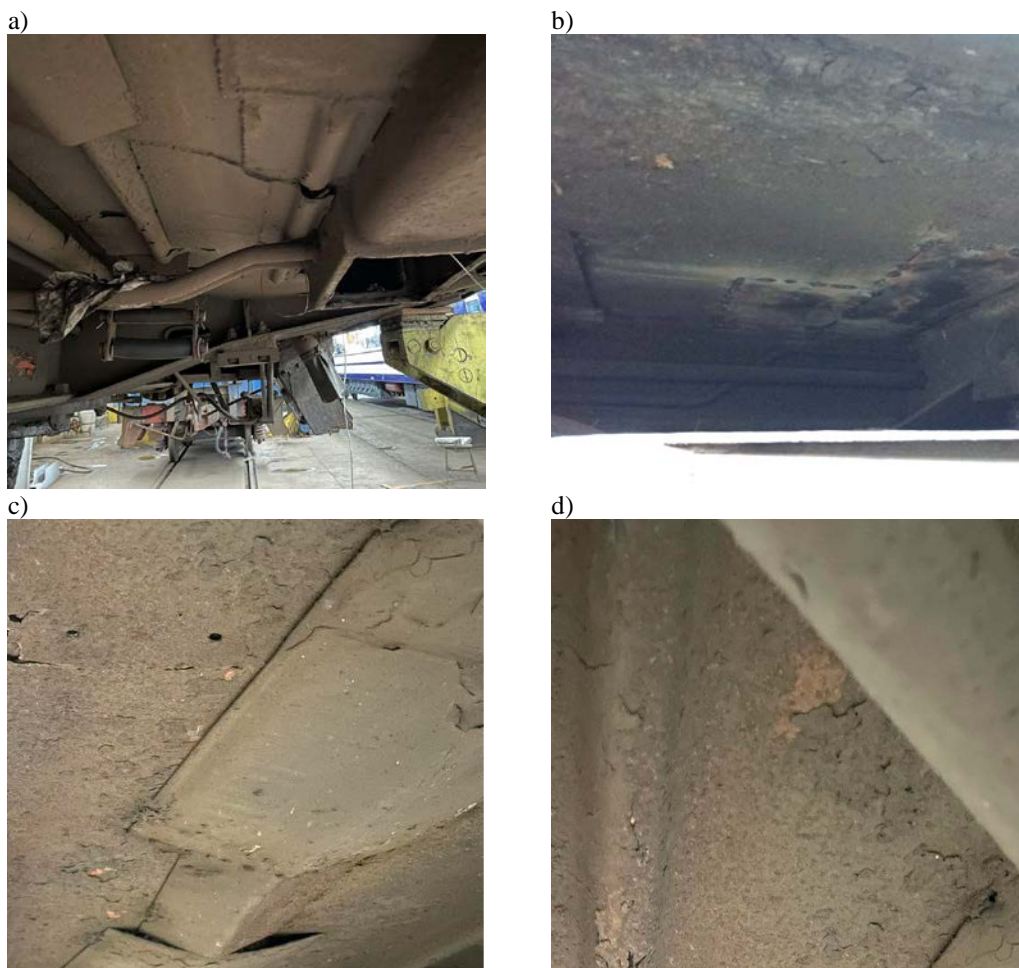
Figure 1: Damage of the main supporting structure of a passenger car - a frame: a), b), cracks of sheets; c) break of the welding seam; d) corrosive wear and cracks
