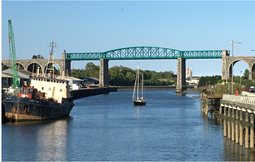
Figure 3: Boyne Viaduct near Drogheda, Ireland. Photo by R. Loendersloot.
